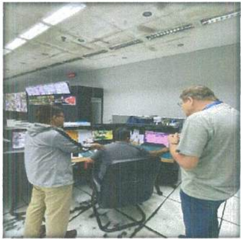
OCC Workstation for SCADA
