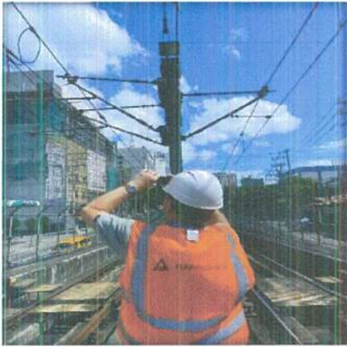
Overhead Catenary System
