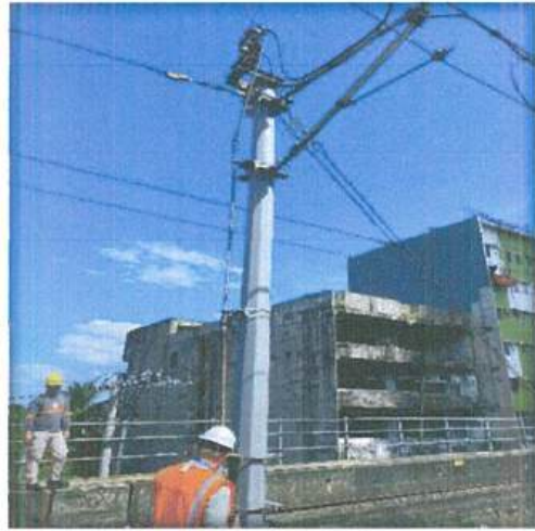
OCS Wayside Area
