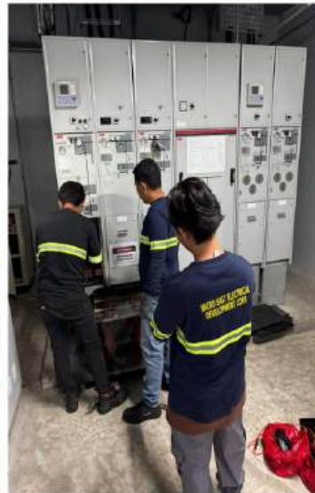
27 February 2026: Negative Tests on 6.6kV RMU at Ninoy Aquino Station, LPS Room conducted by LRTA-PMO, LRMC and BYTP
