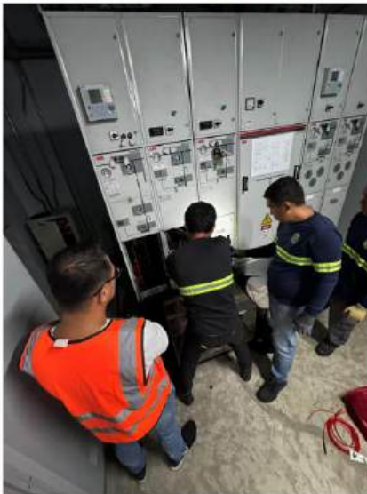
27 February 2026: Negative Tests on 6.6kV RMU at Ninoy Aquino Station, LPS Room conducted by LRTA-PMO, LRMC and BYTP
