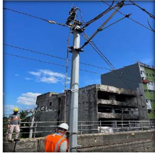
OCS Wayside Area
