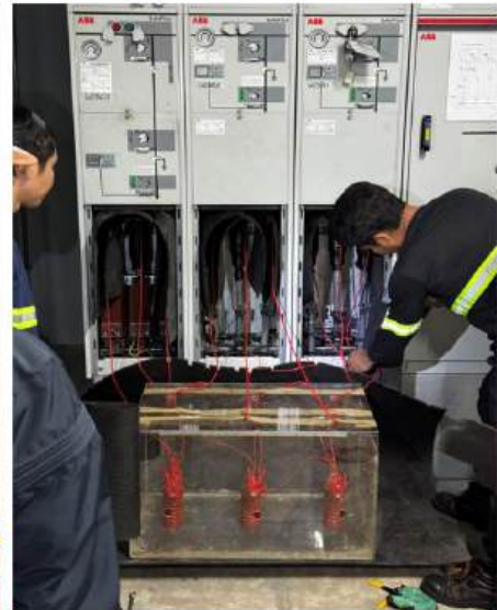
27 February 2026: Negative Tests on 6.6kV RMU at Ninoy Aquino Station, LPS Room conducted by LRTA-PMO, LRMC and BYTP
