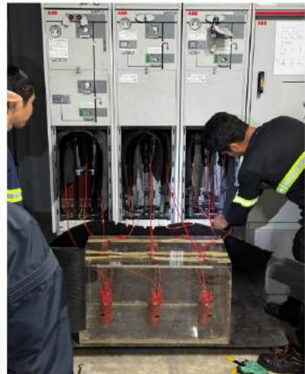
27 February 2026: Negative Tests on 6.6kV RMU at Ninoy Aquino Station, LPS Room conducted by LRТА-PMO, LRMC and BYTP
