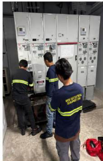
27 February 2026: Negative Tests on 6.6kV RMU at Ninoy Aquino Station, LPS Room conducted by LRТА-PMO, LRMC and BYTP
