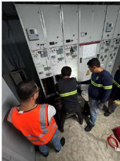
27 February 2026: Negative Tests on 6.6kV RMU at Ninoy Aquino Station, LPS Room conducted by LRТА-PMO, LRMC and BYTP
