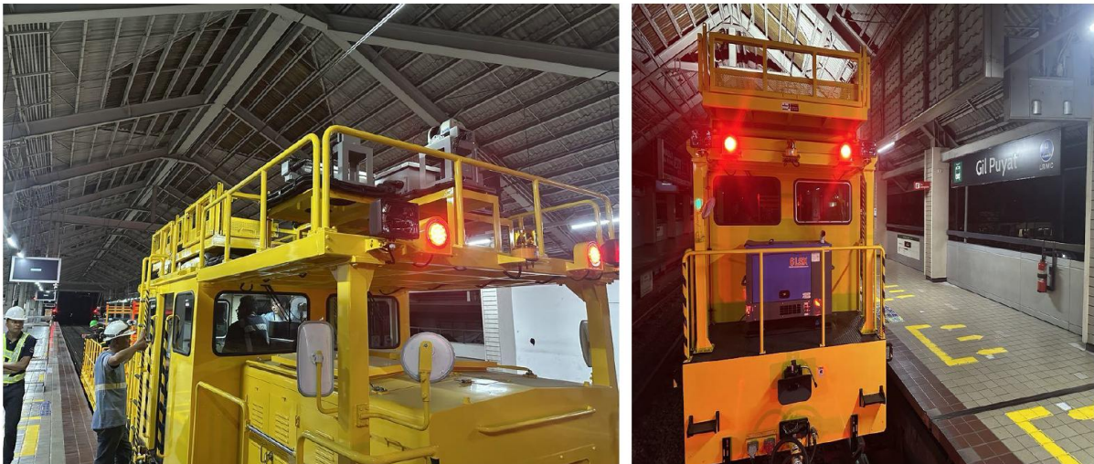
19 March 2025: Practical Training of OCS Inspection System (OIS) represented by LRТА-PMO, LRMC, CMX and YASHIMA Contractor
