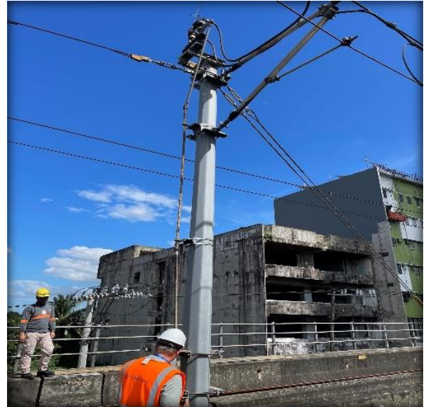
OCS Wayside Area
