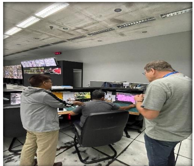
OCC Workstation for SCADA
