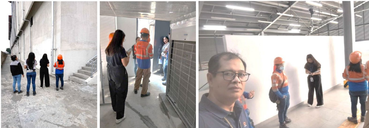
27 January 2025 : Inspection and Validation of Rectified Punchlist Items of the LRT-1 Cavite Extension – Phase 1 Stations with LRMC, EPCC and LRTA-PMO
