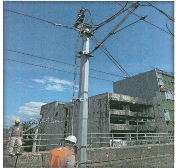
OCS Wayside Area
