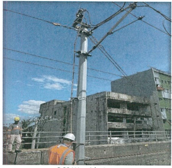
OCS Wayside Area
