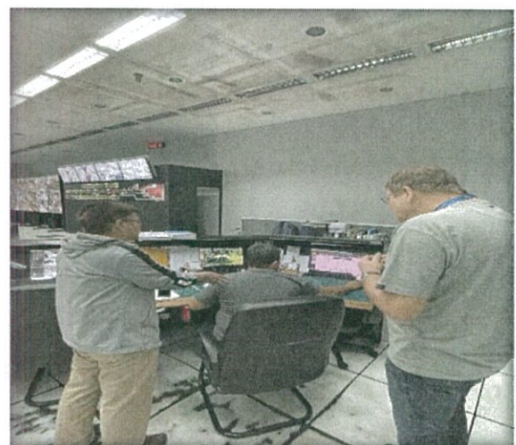
OCC Workstation for SCADA
