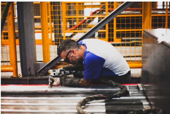
12 December, 2023: Laser Welding Works of G4 Trainset 11 at Baclaran Expansion Depot, Pasay City.
