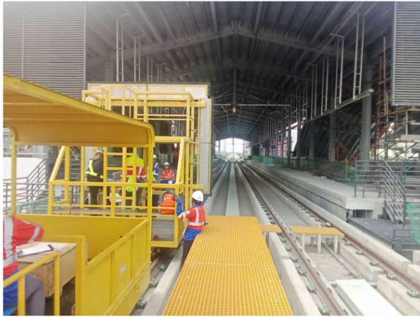
11 December 2023: System Structural Gauge Testing of CEW-ROW P1 using Gauge Trolley.
