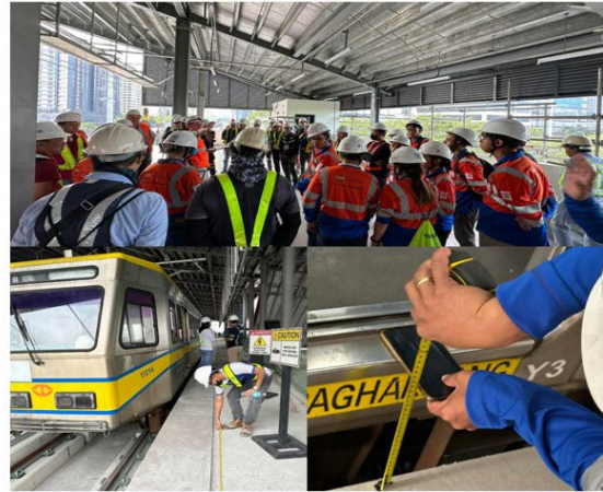
19 December 2023 System Structural Gauge Testing of CEW-ROW P1 using 2 nd Generation Train
