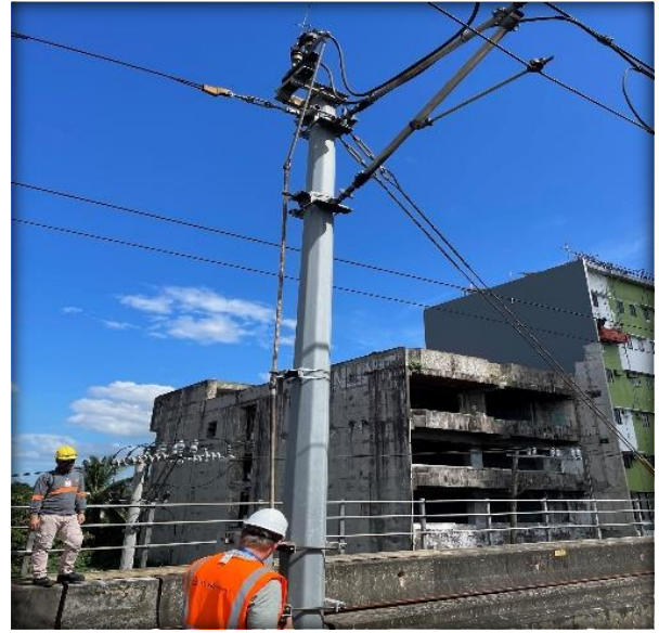
OCS Wayside Area
