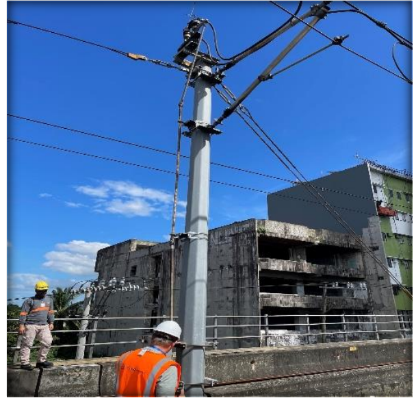
OCS Wayside Area
