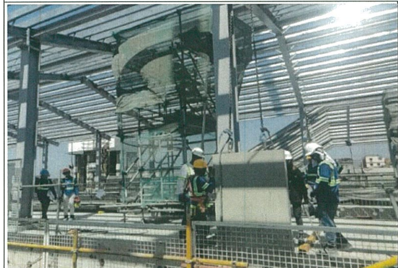
Precast Panel Installation Works in Dr. Santos Station
