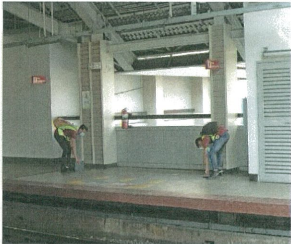
VERIFICATION OF COLUMN DISTANCES AT QUIRINO STATION
