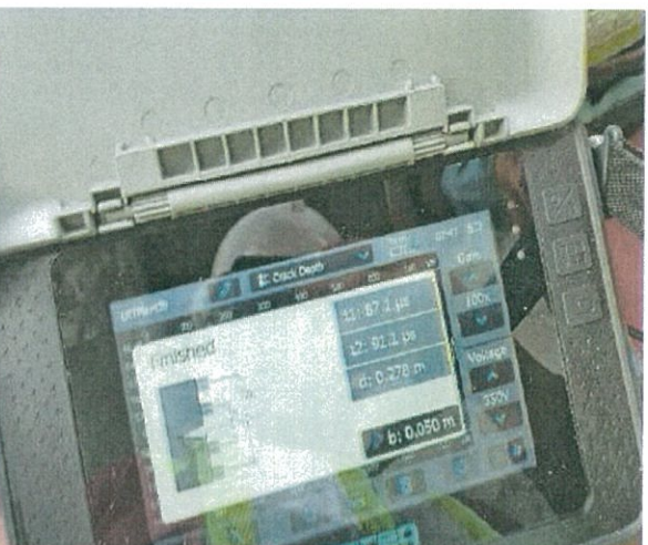
CRACK DETECTION ON COPING BEAM USING ULTRASONIC PULSE VELOCITY TEST
