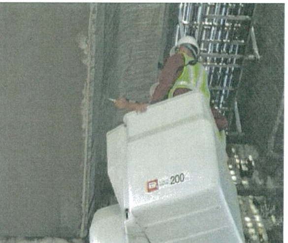
REBOUND HAMMER ON VIADUCT GIRDER
