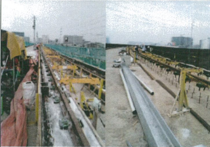
Track works- Rail Tracks Installation
