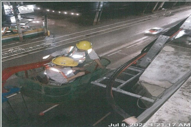
Installation of Additional Cable Tray for OCS Aluminum Feeder Cable
