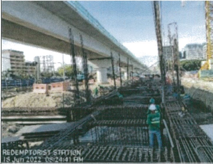
Rebar and Formwork Installation in Redeptorist Station
