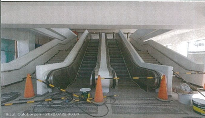
On-going construction of Antipolo Station Eastbound Access Stairs
