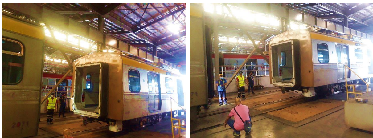
Photo by Engr. Jovito Carino during the ongoing repair/restoration of Trainset Nos. 18 and 13
