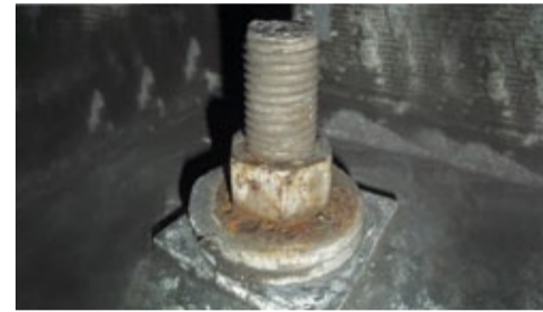
Corroded Anchor Bolts have to be replaced.
