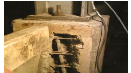
Corroded Anchor Bolts have to be replaced.
